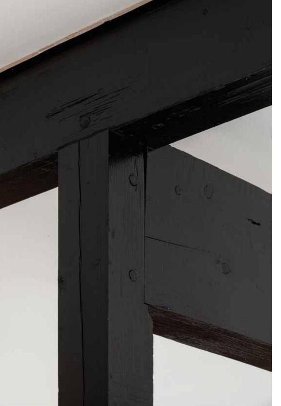
The main constructive principle of the house is a three-dimensional purlin system of black-painted pine.
