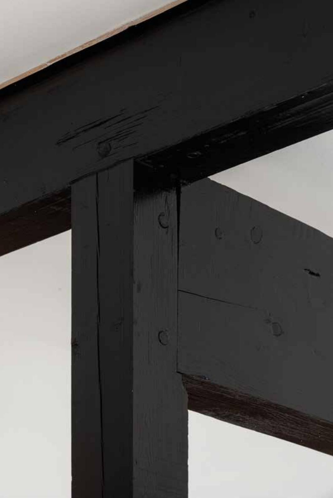
The main constructive principle of the house is a three-dimensional purlin system of black-painted pine.
